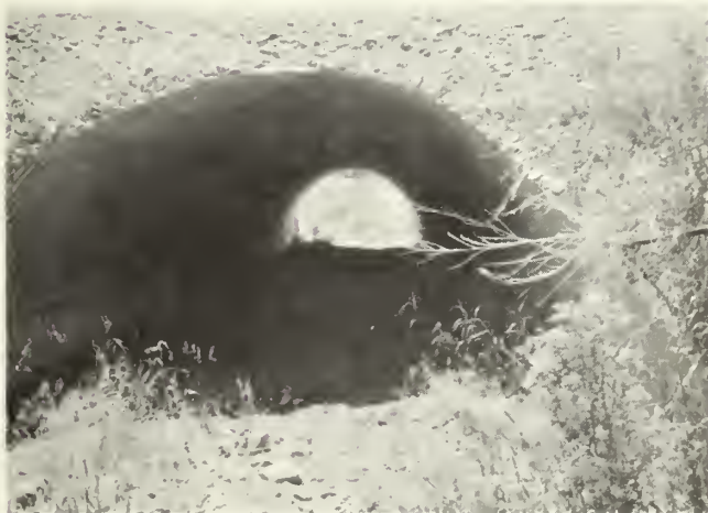
North End of Pipe
